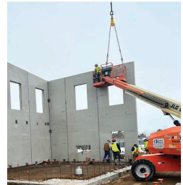
Progress is happening at our Sioux Falls office expansion.
