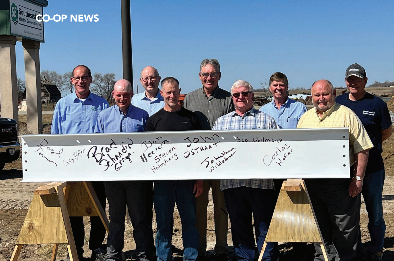
General Manager Brad Schardin and SEC Board of Directors signed a “signature beam” that will be used for a structural beam for the Sioux Falls office expansion. L-R: General Manager Brad Schardin, board members: Sec., Johnathan Wildeboer, John Ostraat, Chris Hofer, Pres., Don Heeren, Treas., Daryl Terveen, VP., Steve Holmberg, Robert Wollmann & Carlos Hofer.
