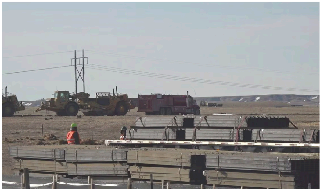
Construction began earlier this year on a large solar farm near New Underwood in Pennington County. Some of the power will be purchased by Basin Electric and be distributed to cooperatives in South Dakota.
