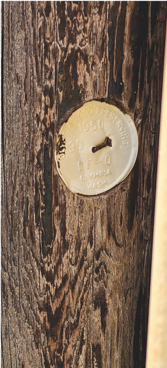
One of the original utility poles on Ken and Kathleen Meier's land was created in 1950, yet it still functions to this day.
