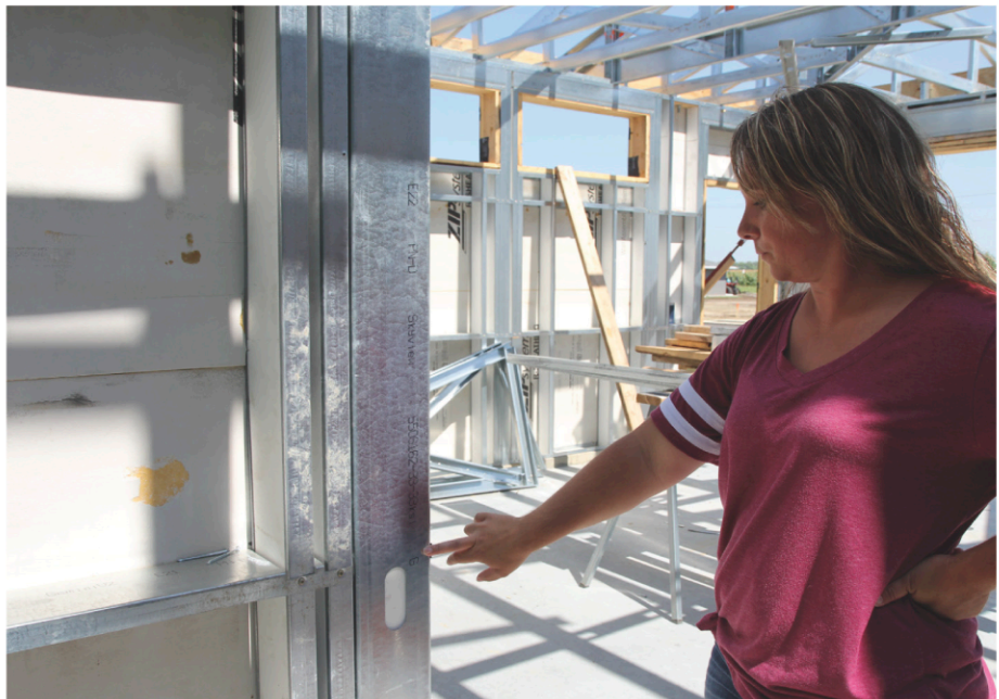
Jackie Adolph points to a label on one of the steel components, which was generated by the design software to ensure the pieces are properly assembled. Photo by Shannon Marvel
