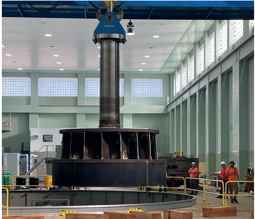
Above: The Fort Randall Dam is equipped with eight turbines. Unit 6 turbine is shown being removed for the first time since it went online in 1955.
